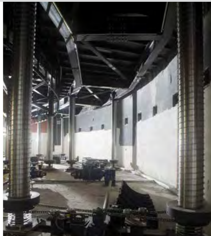
Mobile orchestra platform with Spiralift system
